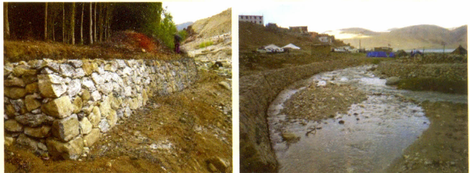
Figure: Soil erosion control measures in different places of Ladakh
