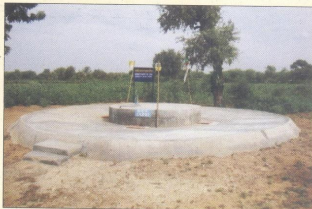
Photo 2. Rainwater harvesting tank
