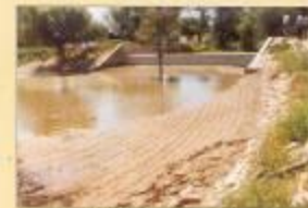
Fig. 11. Khadin system of water harvesting for crop production
