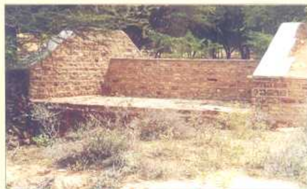
Masonry anicut to control flow of water in an active stream at Jhanwar watershed
