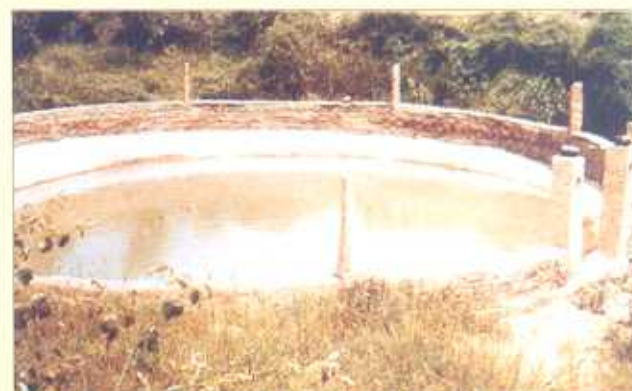
An open tanka of 271 m 3 capacity at farmer's field in Jhanwar watershed
