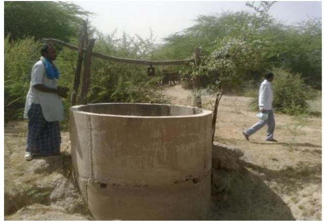
A well made of cement concrete rings in the place of old and abandoned *Virida*
