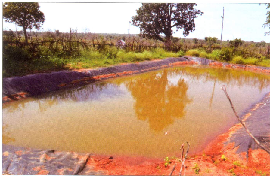
OFR with capacity of 600 m 3
